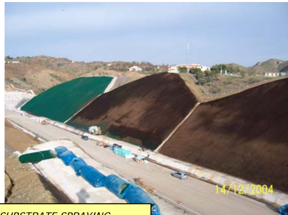
4. SUBSTRATE SPRAYING
